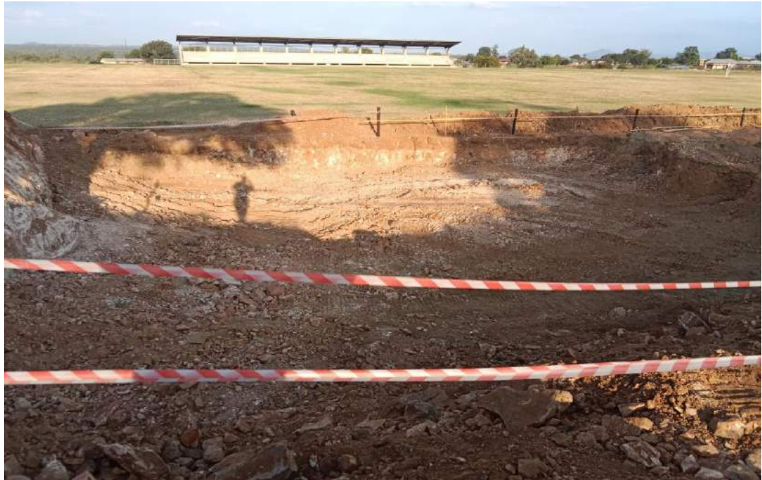
Picture 13 Construction of Davhana Stadium Phase 1
