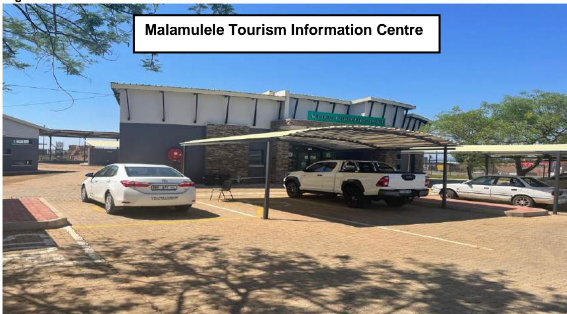
Construction of Malamulele Tourism Information Centre
