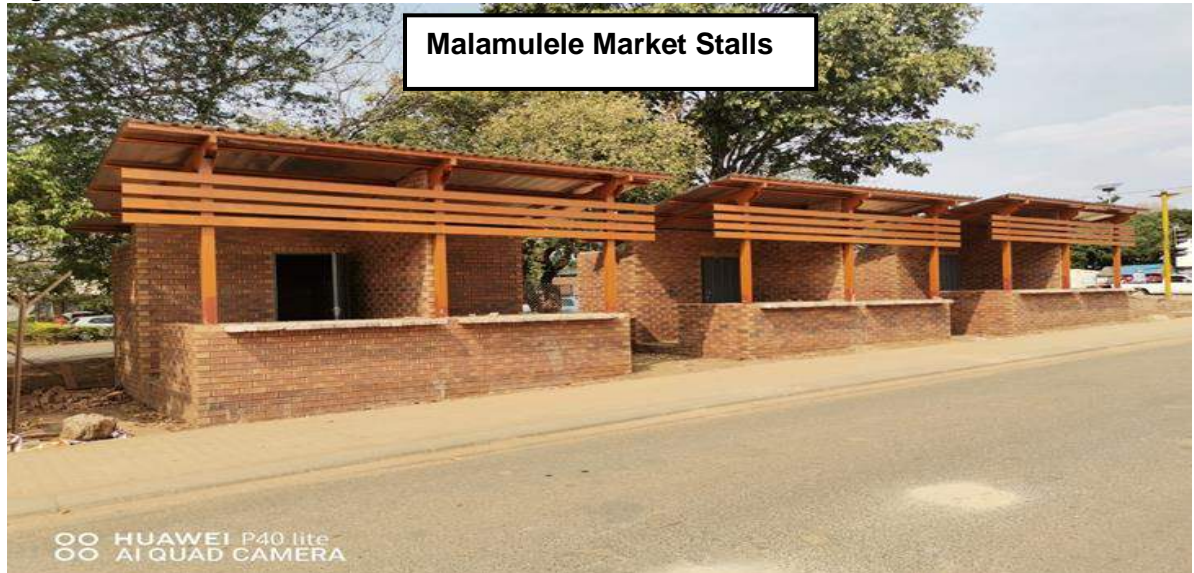
Construction of Malamulele Market Stalls
