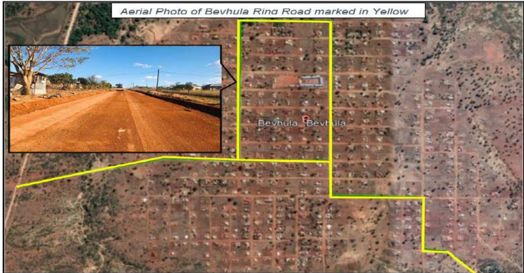
Picture 8 Upgrading of Bevhula Ring Road.
