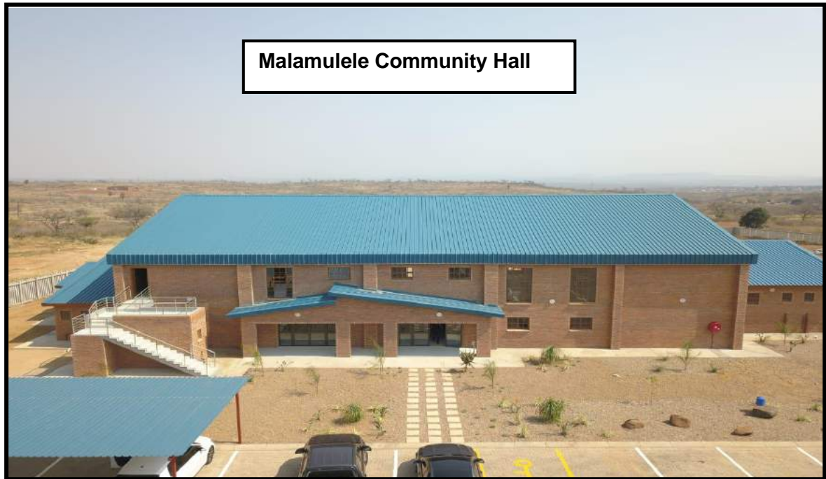
Construction of Malamulele Community Hall
