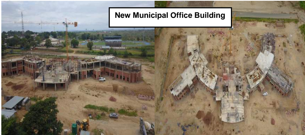
Construction of New Municipal Office Building
